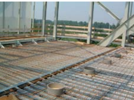
Composite slab used in the auditorium area
