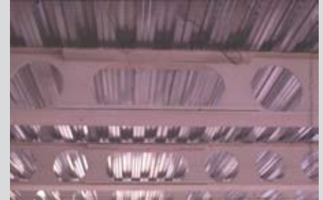
Figure 2.2 Elongated openings in beams with horizontal stiffeners
