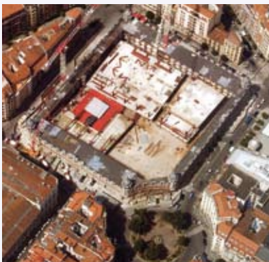
Top view of the construction site (May 2006)
