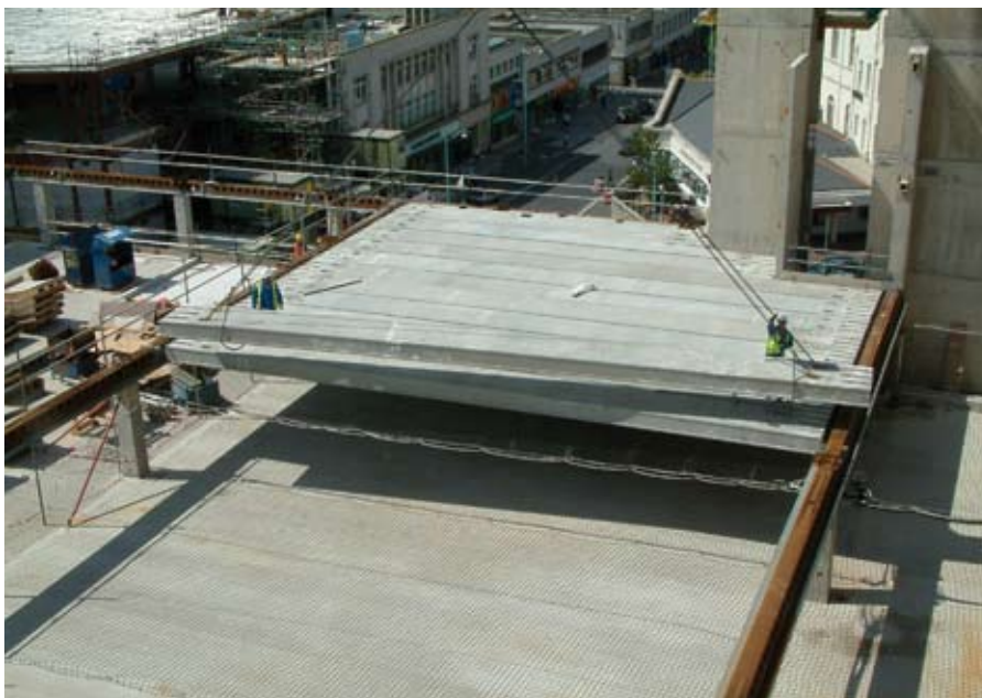
Figure 3.15 Precast concrete units placed on non-composite beams
