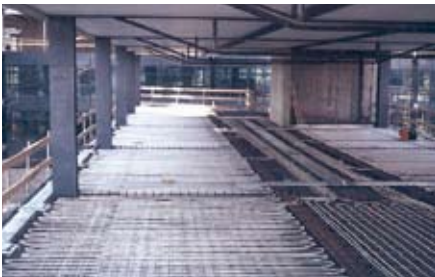
Water heating/cooling pipework placed within the floor slab
