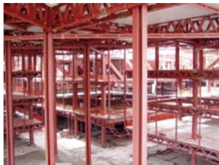
Steel structure of the main entrance hall in front of the cubes
