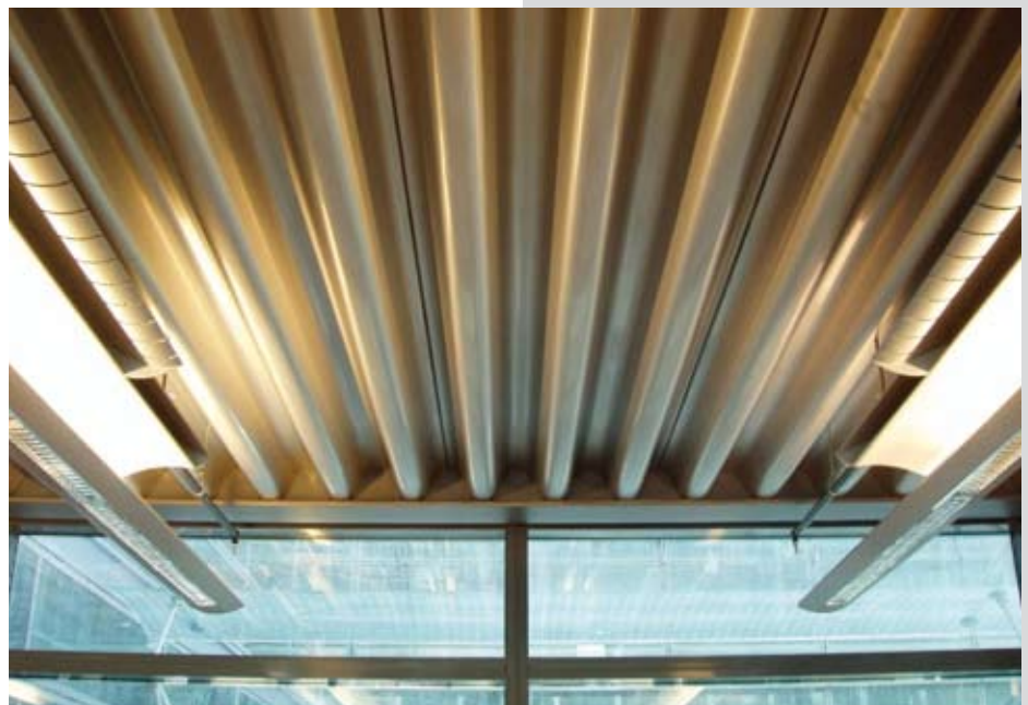
Figure 2.4 Stainless steel composite decking used at the Luxembourg Chamber of Commerce Vasconi Architects
