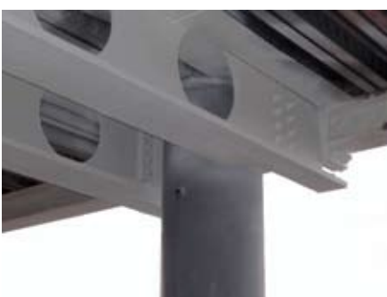
Tubular column connection
